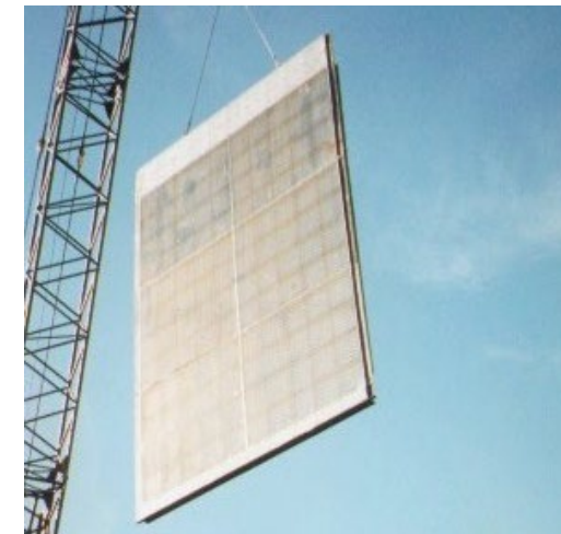
Fish Diversion Flat Panel
